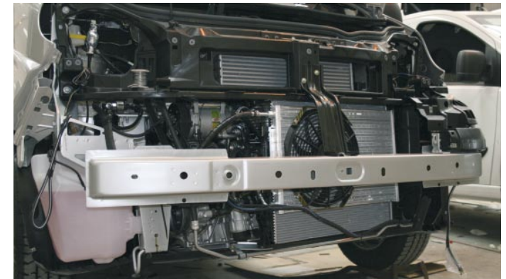
Under-bonnet condenser unit being fitted inside the engine bay
